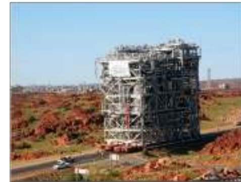
Above: Woodside LNG V module being transported to site during construction
